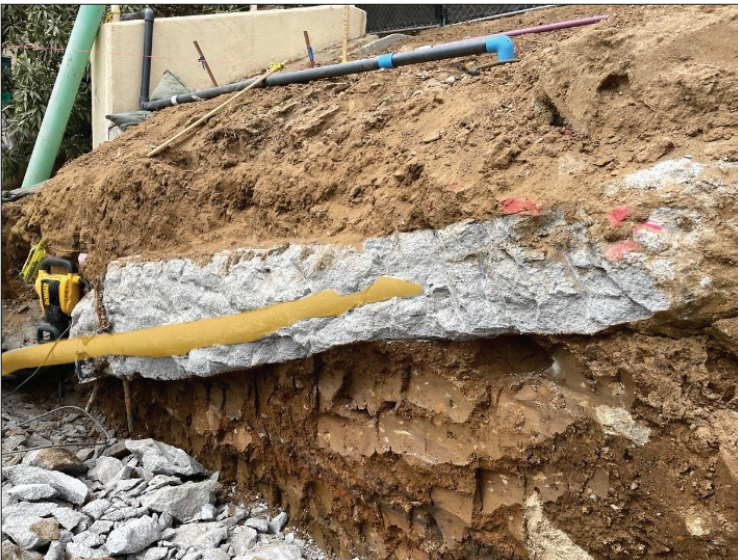
A. Photo of exposed utility for collection
