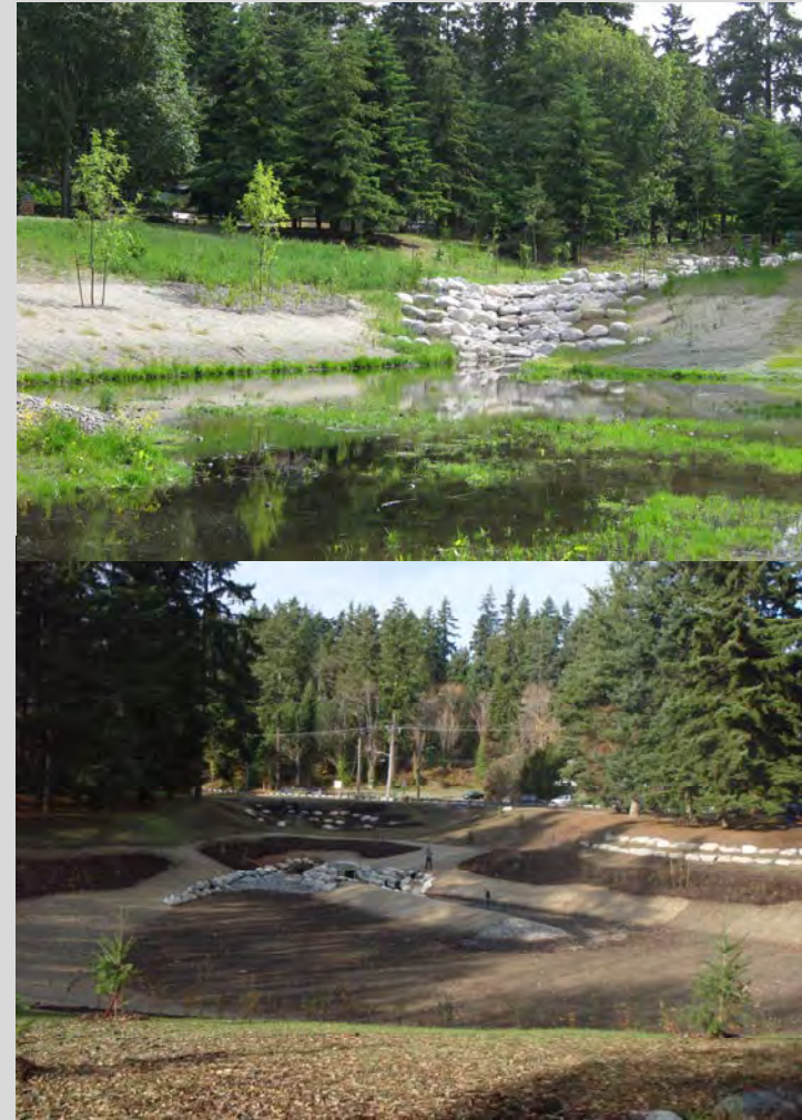
Boeing Creek Park Stormwater Detention/Infiltration Pond, City of Shoreline
